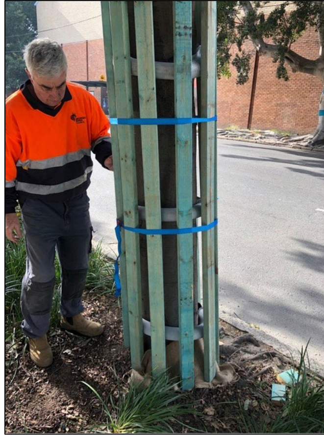
Finished trunk guard with hessian or carpet over buttress/base of tree. Poly plastic strapping.
