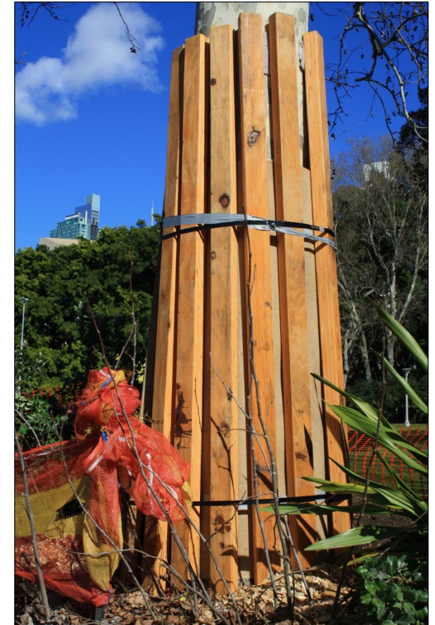
Timber tree guard with thick carpet beneath to cushion trunk from direct contact with battens or external impacts. Galvanised hoop strapping.
