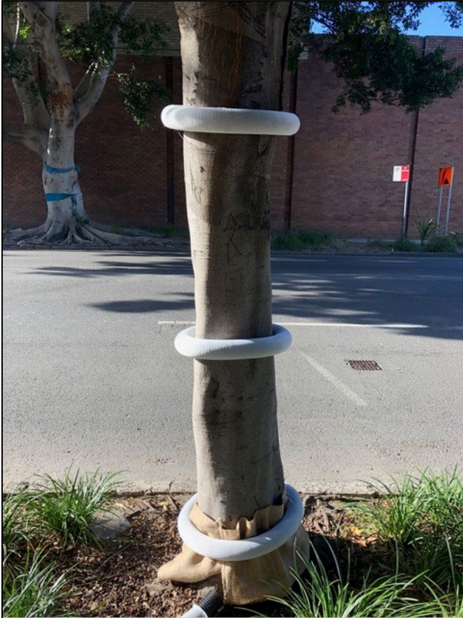
Agricultural pipe with sock to provide cushioning before placing timber battens.
